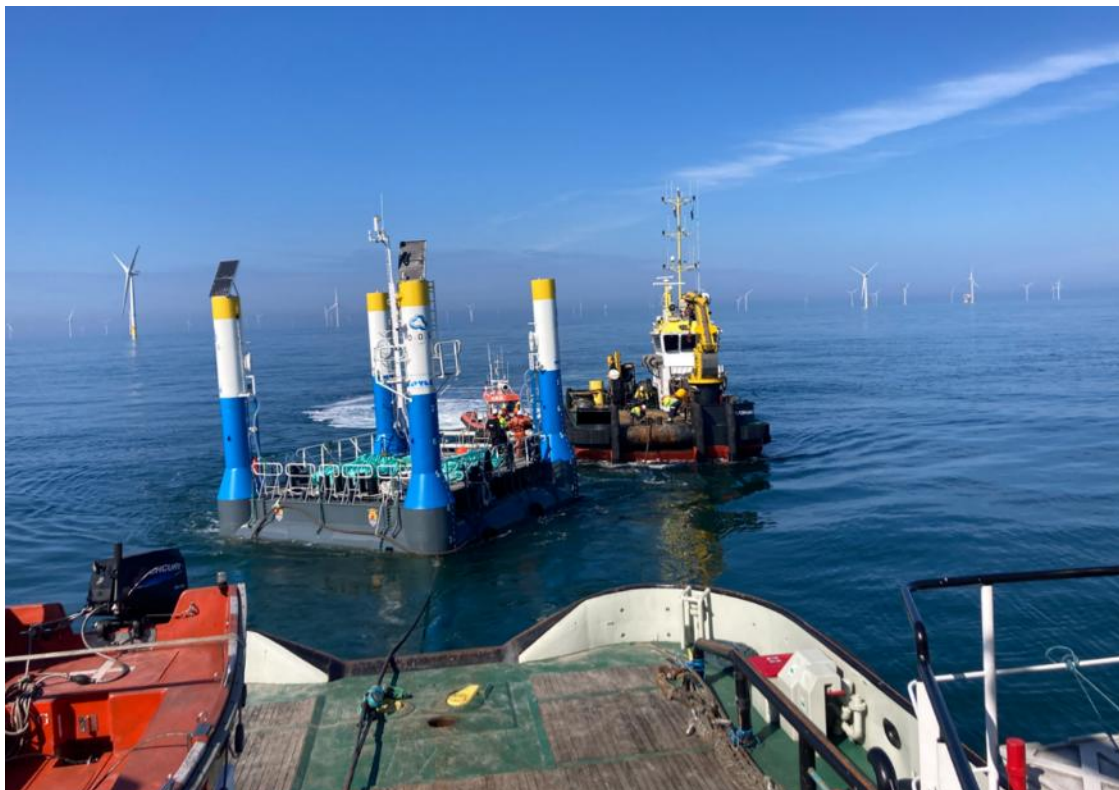
Figure 14. Dutch pilot. Top: Towing and installing the OOS platform in windfarm Borssele (photo OOS).
