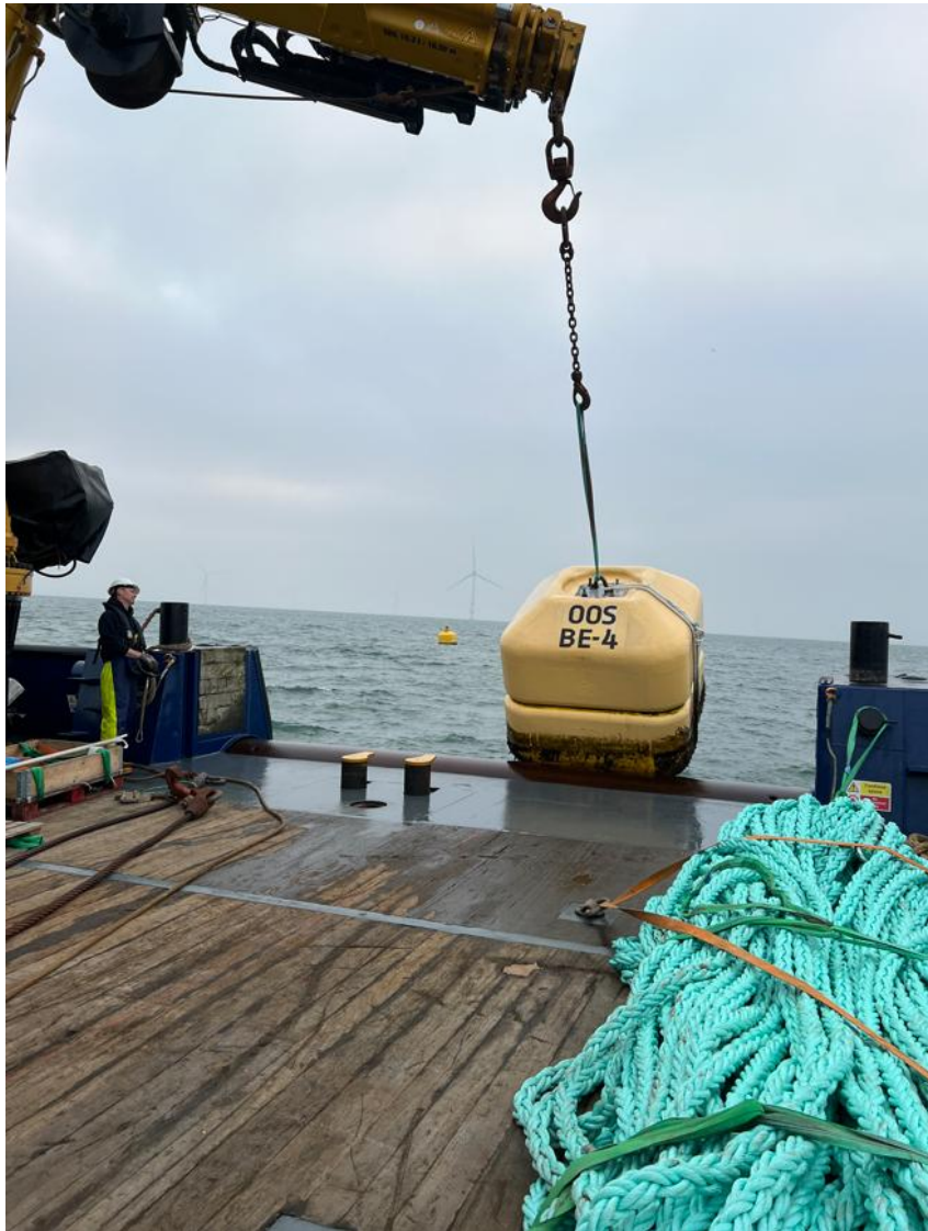
Figure 15. Dutch pilot. Installing end-buoys (photo: OOS).
