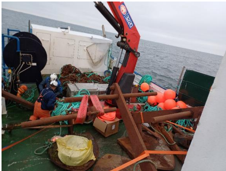
Figure 17. Danish pilot - Anchors and chain on board Frigg ready for installation on the farm.
