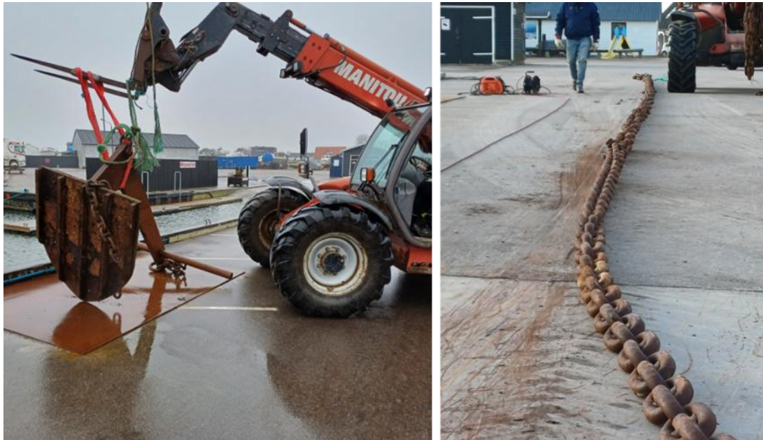
Figure 16. Danish pilot – preparation of anchors and chain on land.
